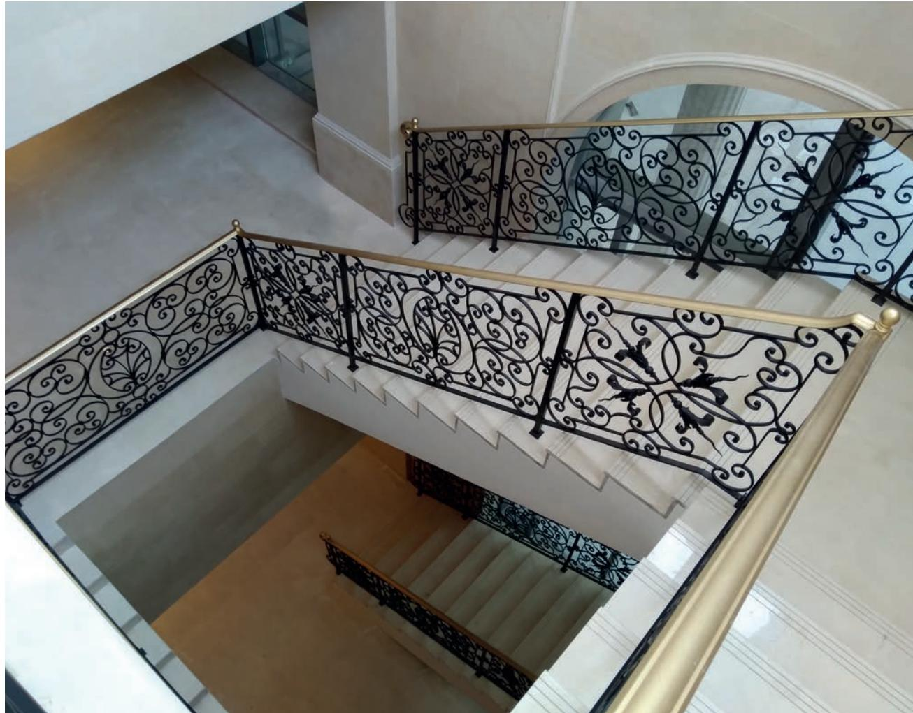
A completely customized project that began with a preliminary on-site study to carefully analyze the installation and stylistic requirements. Our in-house designers then developed sketches for the original decorations, from which all the painted iron and brass elements that make-up the railings were handcrafted in Italy. Brass was chosen as the material for the handrails, a solution that gives a precious shine to the main staircase that majestically welcomes guests from all over the world.
