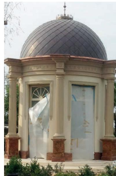
Details of the shingle coverings in teku oxid
