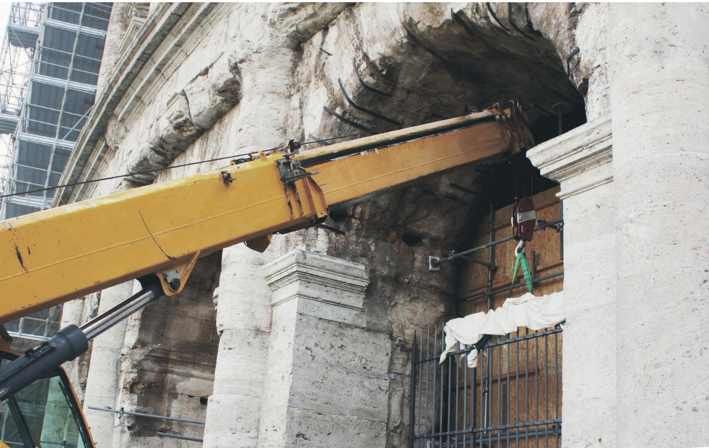
The total weight of the products and the dynamics of the positioning required the use of special vehicles. In these photos a detail of the dynamics of the laying works is represented. The gates, after being positioned, have been set by our team of experienced installers.
