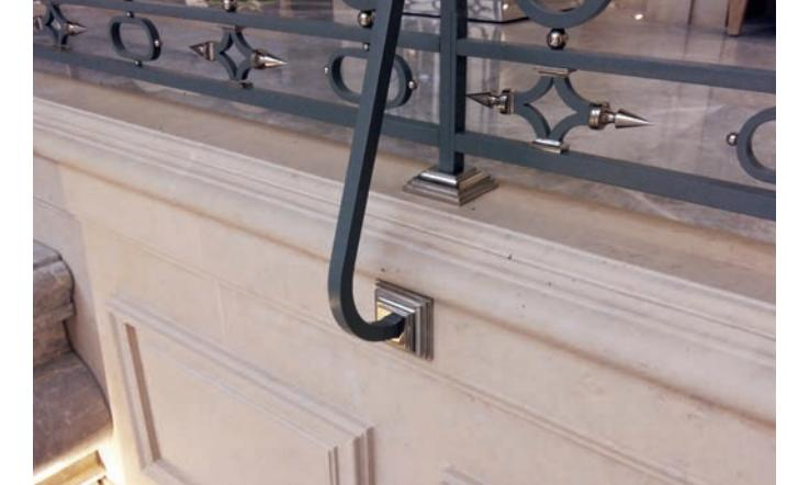
Detail of fixation elements of balustrades on floor and on wall
