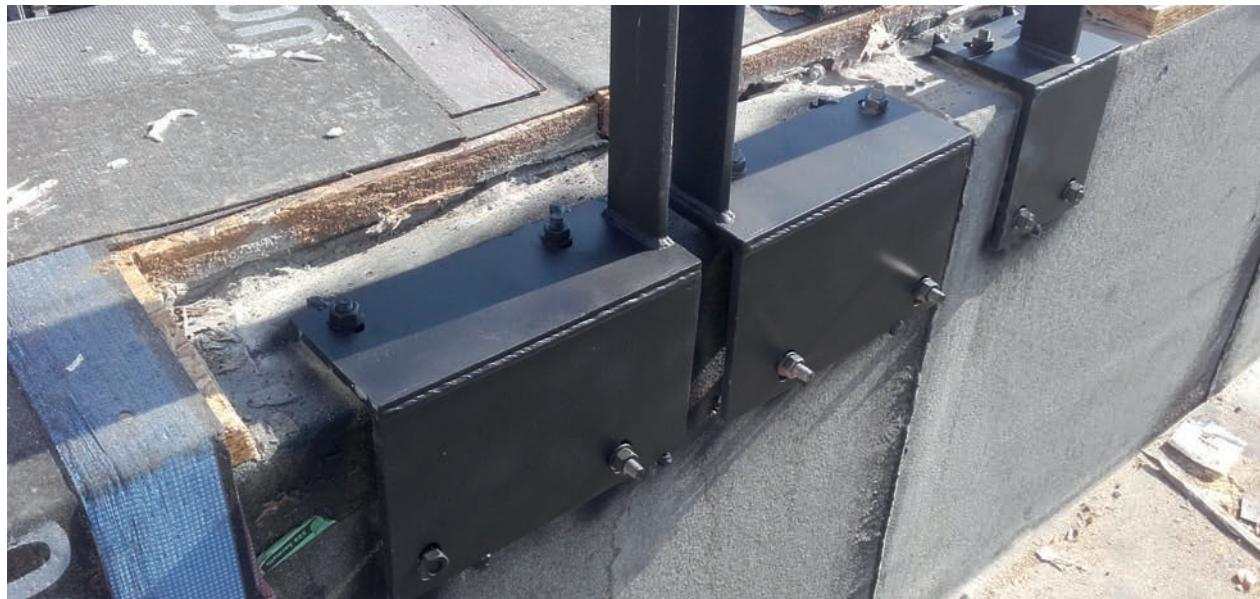
Detail of the bracket specially designed for public spaces. It is able to resist the 3kN/m load
