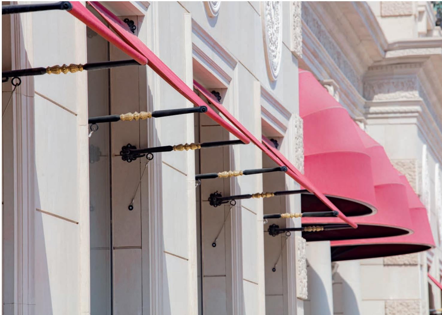
This picture shows a perspective view of the external arms awnings and basket awnings. Both support systems have been studied and designed to be resistant to sandstorms, typical of Qatar area. Structure is in aluminium and decorative parts are in painted wrought iron with brass elements.
