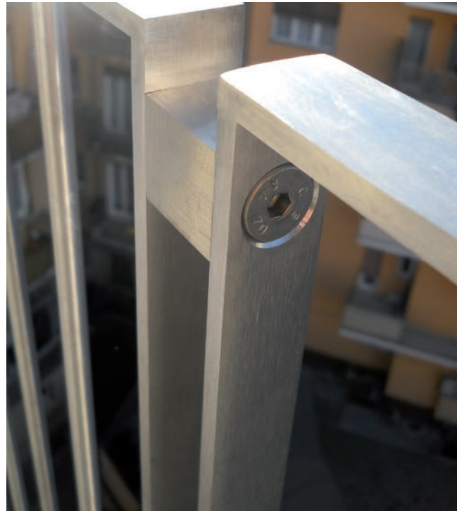
Detail connection of infill panels Dettaglio connessione pannelli tamponamento
